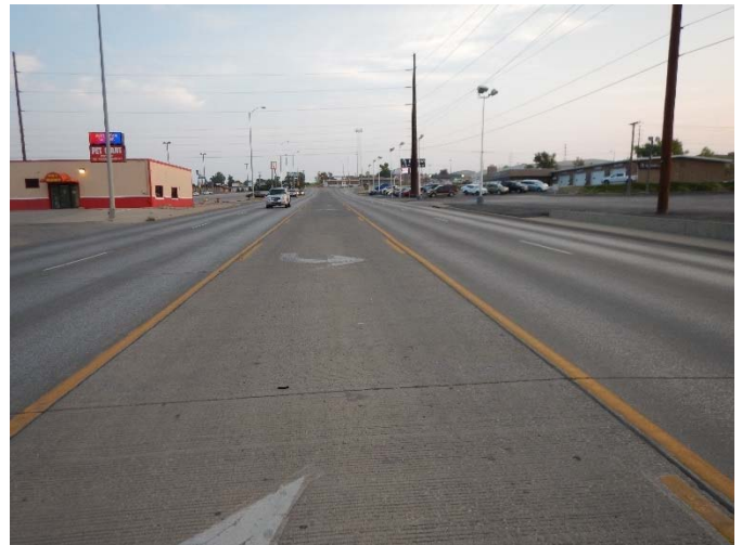
Figure 1.4 – Pavement on Cambell Street
