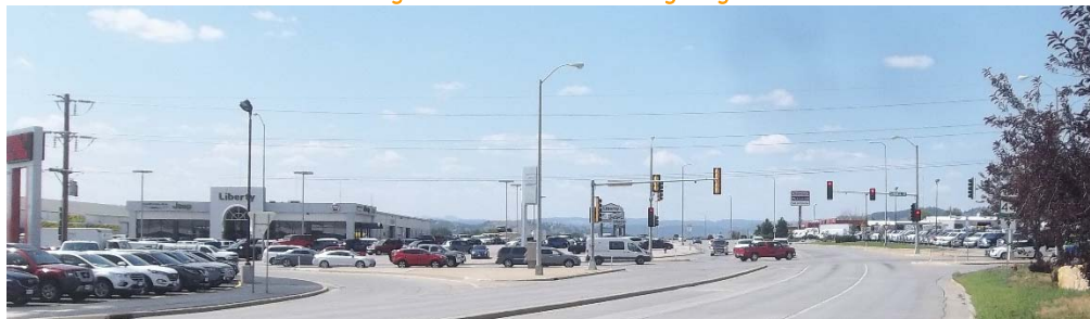
Figure 1.7 – Omaha Street Lighting
