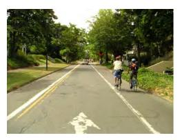
This contraflow bike lane in Portland, OR (left) provides a key connection along a narrow one-way street.
