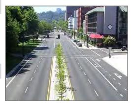
This street previously had 13' lanes, which were narrowed to accommodate bike lanes without removing a lane.
