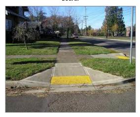
Example of an ADA-compliant perpendicular curb ramp
