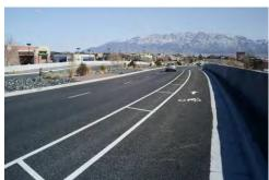
Buffered bike lanes protect cyclists from fastmoving traffic
