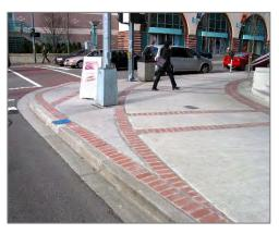
Figure 59. Reducing the radius of a turn reduces traffic speed and greatly improves safety for bicyclists and pedestrians
