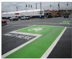
Figure 58. Bike boxes have been installed at several intersections in Portland, OR where right-turning motorists conflict with through bicyclists.
