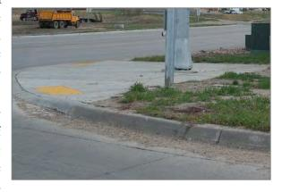
Figure 7. ADA-compliant curb ramp with tactile domes.
