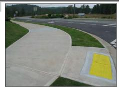
A diagonal curb ramp with detectible warning.
