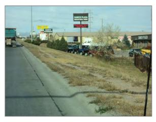
Figure 8. Frequent pedestrian use along Deadwood Avenue is evident by the worn "demand trail", indicating a good location for a pedestrian facility investment.
