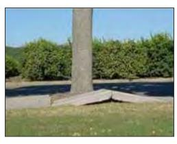
Subsurface tree roots can lift concrete sidewalk slabs, causing the surface to become uneven.
